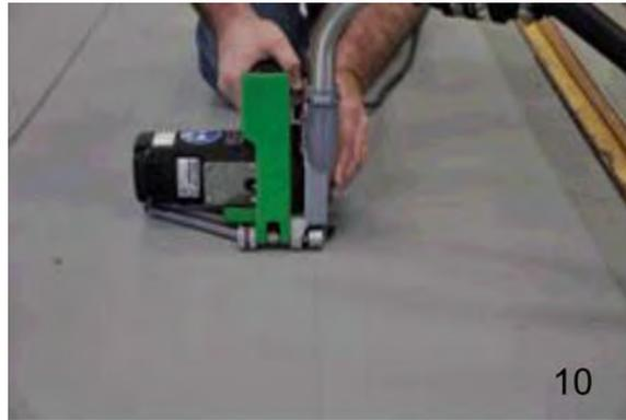
Grooving should be performed so that both sides of the seam have been grooved equally and uniformly- **Image 11.**
